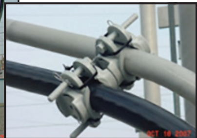
Three-in-one HPI-CRI-U suspended from a Unistrut
