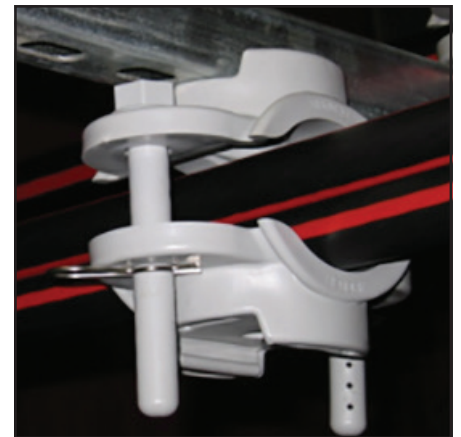
Three-in-one HPI-CRI-U suspended from a Unistrut
